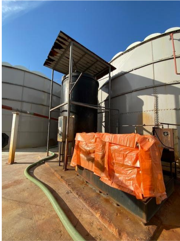
Figure 6: Ferric Chloride storage tank
